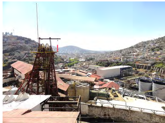
Fig. 9: The San Juan Pachuca mine und Loreto Ore processing (Photo: ESCAMILLA-GONZÁLEZ, 2013)
