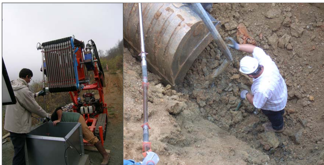
Fig 1, 2: DMS column installation (28 th October 2008) and removal (13 th July 2009) – Bagnaschino site.
