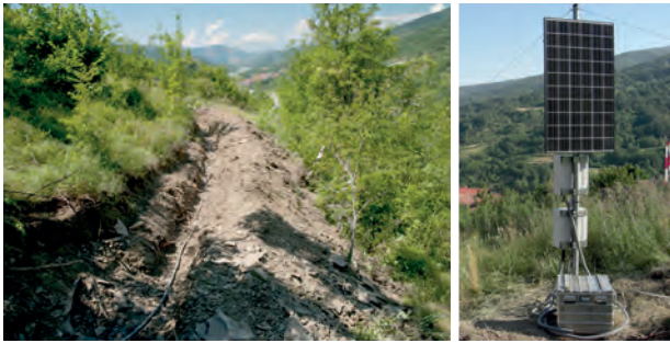
Text-Fig. 2. Installation of the geoelectrical profile (left side); solar panel and „methanol fuel cell“ (right side).
