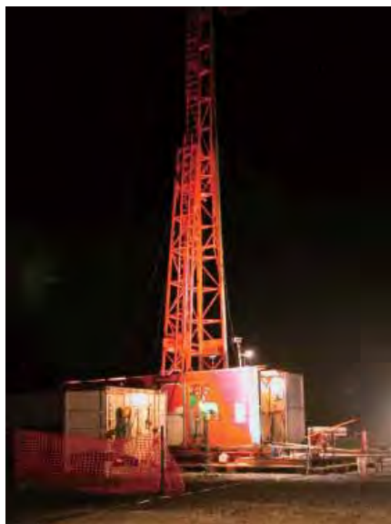
The Chesapeake Drillsite at night.
