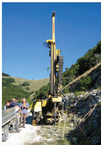
Figure 3. Drilling operations at Poggio le Guaine.
