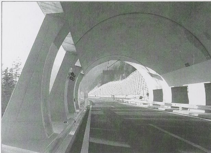
Tunnel for motorway and stabilization of embankments
