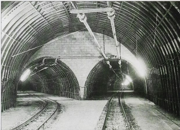
Main haulage level
