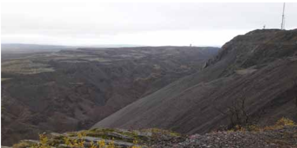
Figure 10: View into the sink holes above the Kiruna orebody
