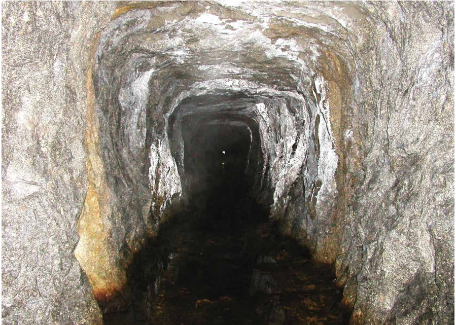
Figure 5.1.2. Interior of the Souš water- supply tunnel in the Jizerské hory Mts. Water runs over the tunnel ground. Klomínský et al. (2005).
