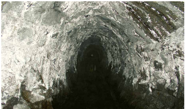
Figure 6.9.1. White opal coatings on walls of the Jizera Granite in the Souš water-supply tunnel. Klomínský et al (2013).
