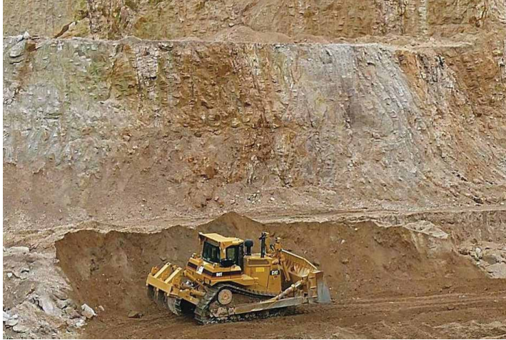
Figure 4.3.2. Tectonic zone of the Sudetic direction in the Liberec Granite, 50 meters wide in construction site near Na Bídě town district (Perštýn locality). Photo J. Klominský.
