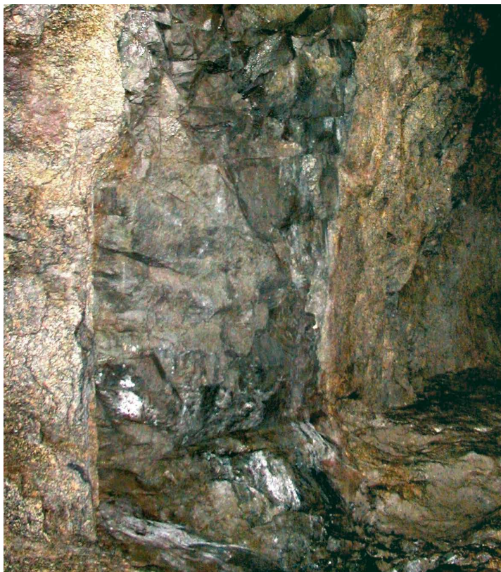
Figure 3.8.1. Trachyandesite dyke 2.5 m wide in the Souš water supply tunnel. Photo J. Klomínský.
