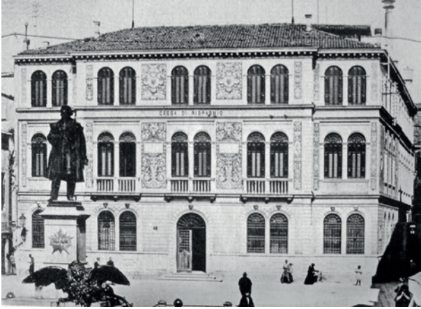
Fig. 10. Venice, main façade of the new headquarters of the Cassa di Risparmio in a photo taken around 1890. Archives of the Cassa di Risparmio di Venezia.
