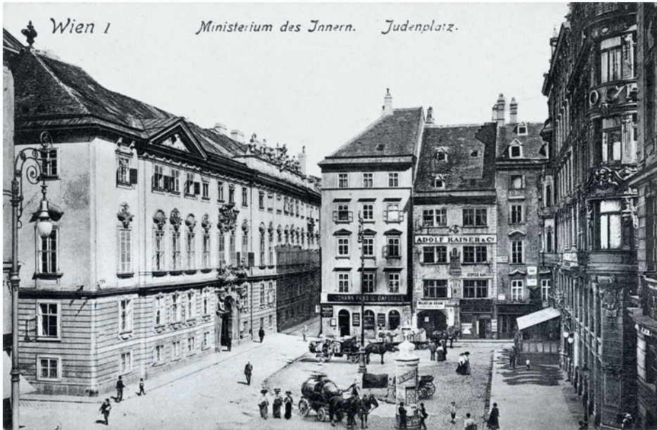
Fig. 2. The façade of the Ministry of Interior in Wipplingerstraße , facing Judenplatz , Vienna, on a postcard of 1910. Photograph by Paul Ledermann. Wien Museum Online collection ID 65861/144 1–3, https://sammlung.wienmuseum.at/objekt/426919-wien-i-ministerium-des-innern-judenplatz/ (accessed 16 April, 2023).
