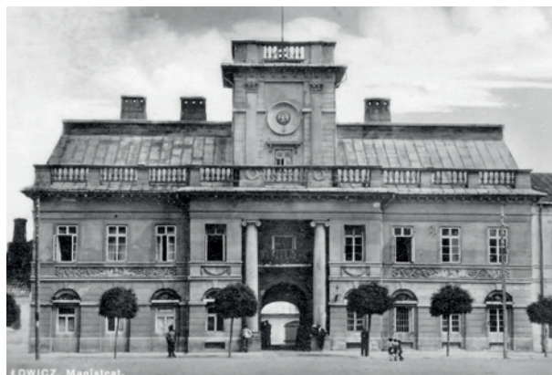
Fig. 8. Municipal hall ( magistrat ) of Łowicz (designed by Bonifacy Witkowski, executed by Jan Trautsolt and Stanisław Perkowski, 1826–31). Early 20th-century photograph in author's collection.
