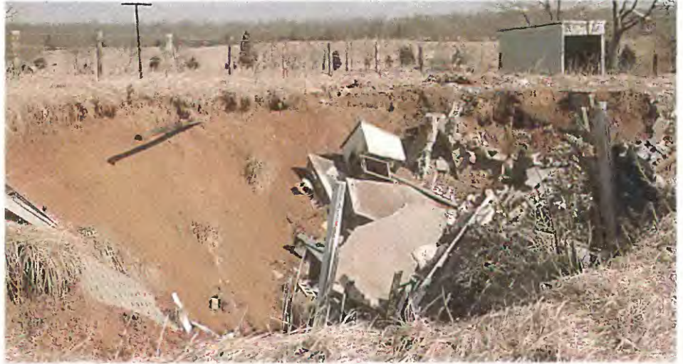
Figure 5. Collapsed home in sinkhole on Ordovician limestone in the Shenandoah Valley exemplifies karst hazards associated with carbonate rocks such as limestone, dolomite, and marble in areas of the Piedmont, Great Valley, and Valley and Ridge. Photo by R.C. Orndorff.
