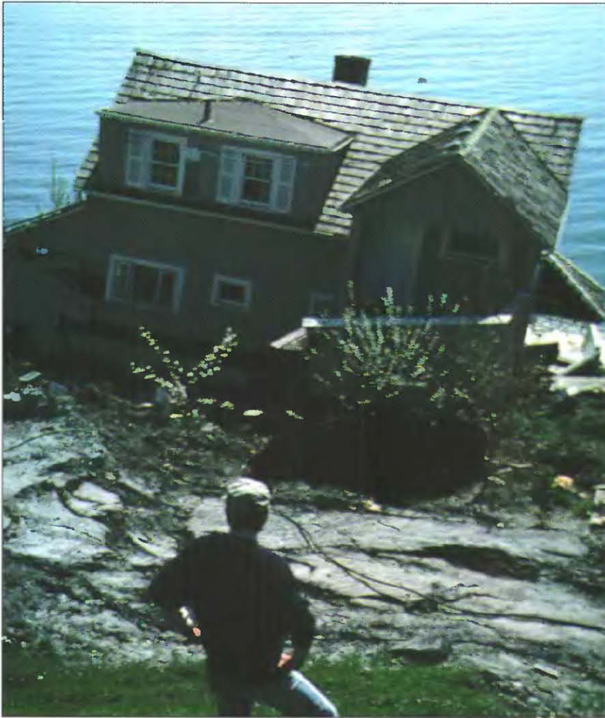
A house (overlooking Puget Sound in the Magnolia area of Seattle) destroyed by a landslide. (Photo: Ed Harp, USGS)
