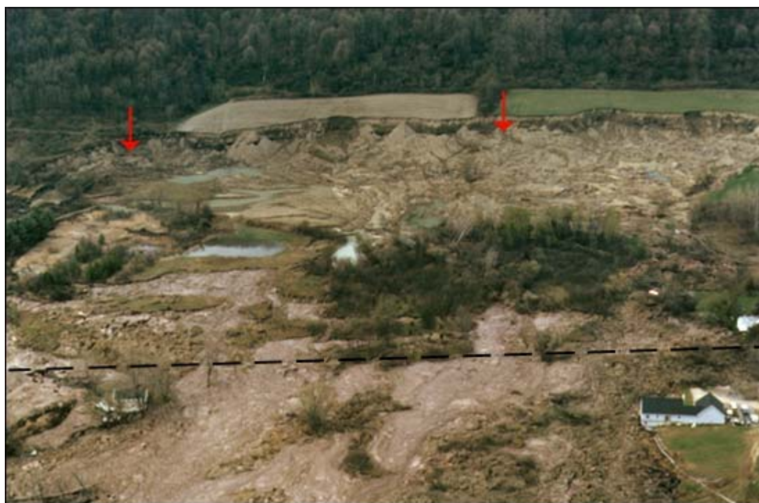
Figure 1. Oblique aerial view of the Tully Valley landslide taken April 30, 1993, 3 days after the slide. Debris moved toward the viewer, in the process covering Tully Farms Road (dashed line) up to 15 feet deep with reddish remolded clay.
