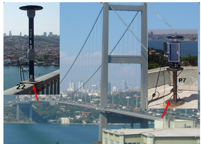
Fig. 2. Reference (P7) and object (22) points used on Bosphorus Bridge during Eurasia Marathon.
