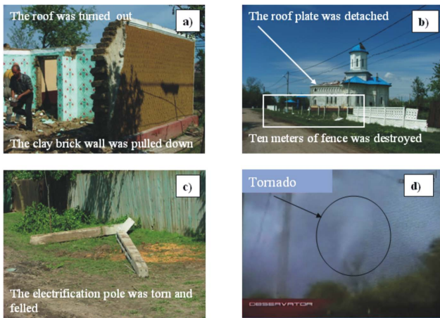
Fig. 4. Damage survey in Movilita village.
