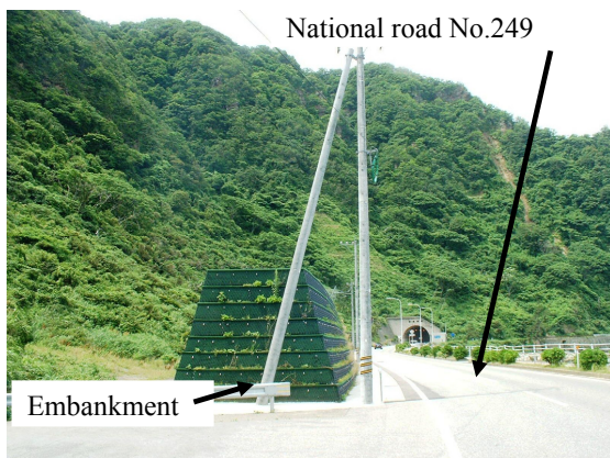
Fig. 14. Constructed embankment against rockfalls.
