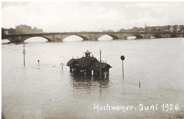
Fig. 1. Picture of the Elbe river extreme flood event in summer 1926, with flood crest on 22 June 1926 and a peak value of 6.98 m above recent gauge datum (private collection M. Deutsch).
