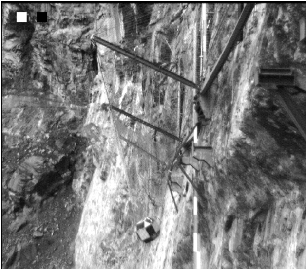
Fig. 5. Photogram of the video of a full-scale test in a vertical test site for a 500 kJ net fence when the maximum elongation is reached (courtesy SAFE s.r.l.).
