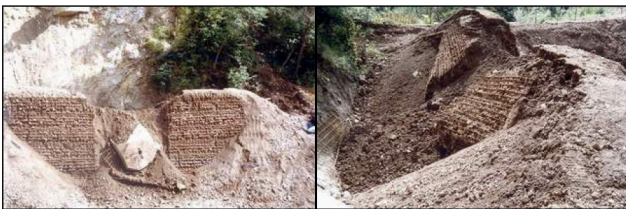
Fig. 4. Unreinforced embankment after the impact in test 3 (Peila et al., 2007).
