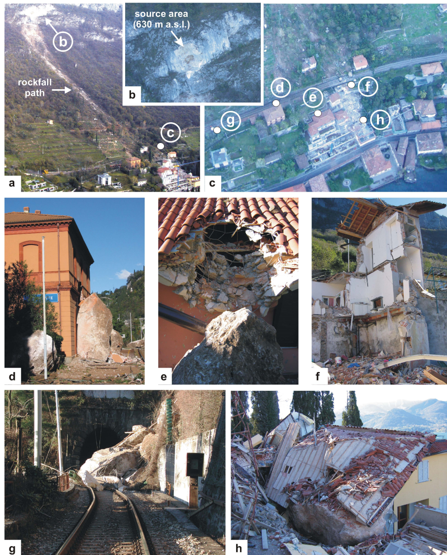
Fig. 2. The 2004 Fiumelatte rockfall event. (a) NW view of the affected area, including rockfall source and path; (b) detail of the rockfall source area; (c) aerial view of the impacted area, including the inner part of the Fiumelatte village, the Lecco-Colico railway track and the SP72 road. Numbers indicate the location of structures in d) to h). (d) railway station (n. 42 in Fig. 8), damaged by the impact of a 30 m 3 block; (e) roof of building n. 46 (Fig. 8) damaged by a 8 m 3 block; (f) three-storey building (A in Fig. 8) destroyed by a 96 m 3 block, where two casualties also occurred; (g) damaged railway section west of the main rockfall corridor; (h) building n. 53 downslope of building A (Fig. 8), severely damaged by the same 96 m 3 block.
