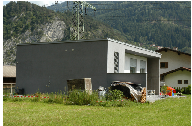
Fig. 23. New building: Strengthened front wall without windows.
