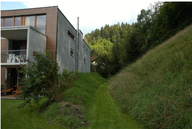
Fig. 22. New building and upgrade: Earth-filled dam for energy dissipation of falling rocks.
