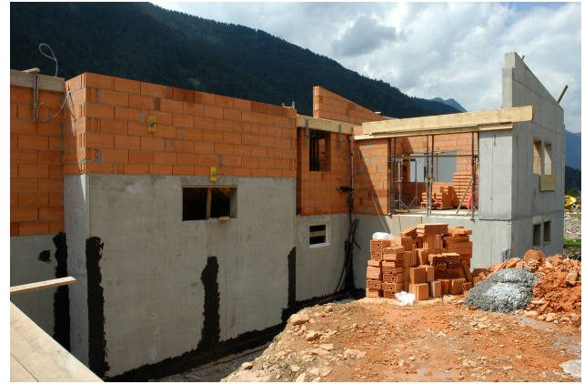
Fig. 2. Brick walls reinforced by ferro-concrete components to strengthen the building's resistance.
