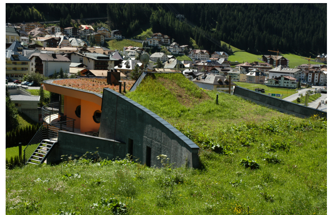
Fig. 28. New building: Roof terrace to integrate the building into the surface of the slope.
