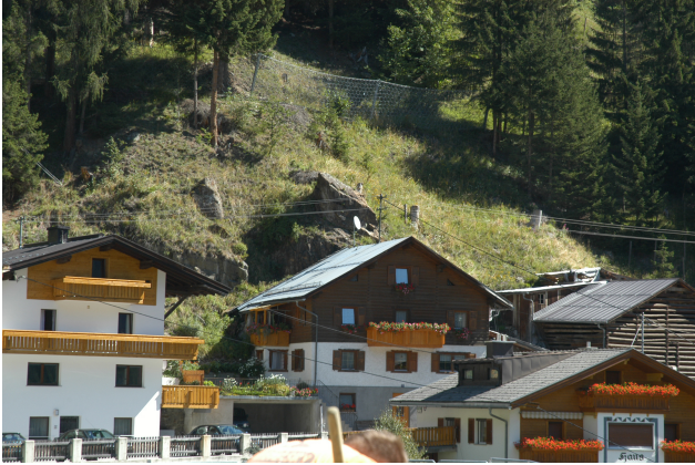
Fig. 24. Enclosing structures: Net barrier to protect buildings against rock fall.
