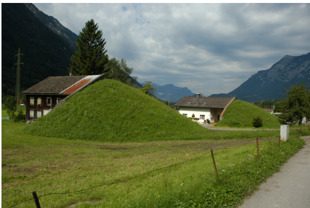
Fig. 27. New building and upgrade: Earth-filled dams as deflection and splitting facilities.
