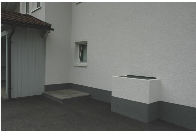
Fig. 9. New building and upgrade: Enhancement (raising) of light wells above flood level.
