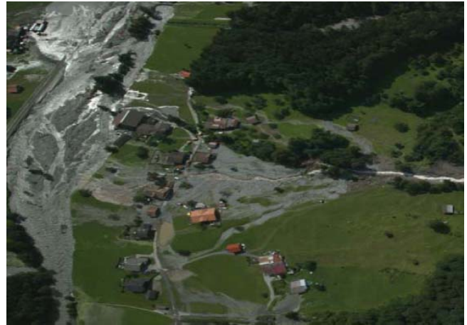
Fig. 3. Deposition cone of Glattbach torrent. Aerial image by Swiss Air Force, August 2005.
