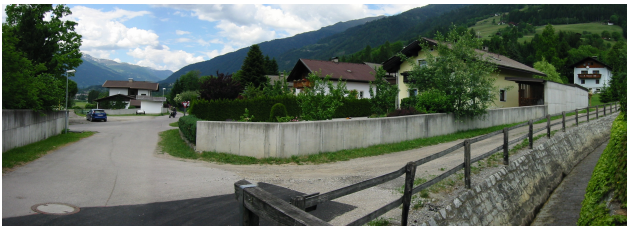
Fig. 5. Local protection measures in the Wartschensiedlung village.
