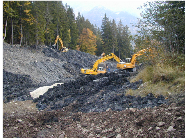
Fig. 12. Execution of deep drain trenches.
