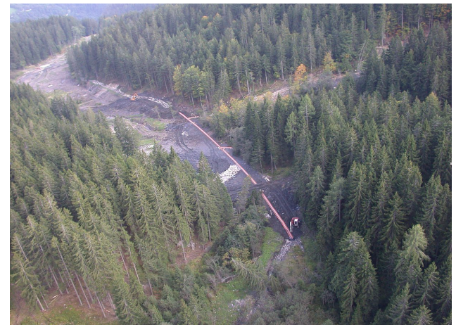
Fig. 10. Executed peripheral surface drainage at the western landslide edge above the prefabricated bridge.
