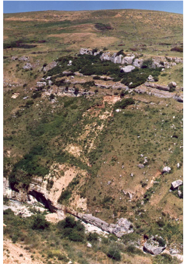
Fig. 2. Shallow translational slide triggered in November 1983, in the East slope of the Trancão valley (Trancão sample area).
