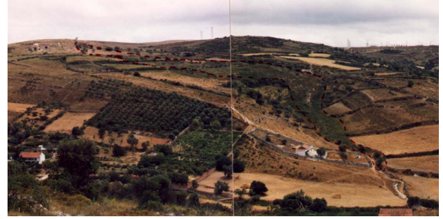
Fig. 5. General overview of the “Quebradas” complex slope movement (Fanhões sample area). The landslide developed in February 1979 as a deep translational slide, evolving downslope to an earth-flow.
