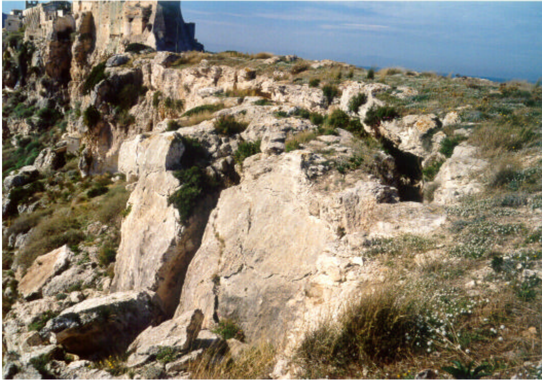
Fig. 8. Secondary toppling mechanism induced by weathering of underlying marly calcisiltites (E side of the Isle of San Nicola).
