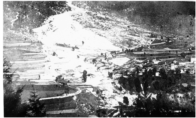
Fig. 4. Damages from the debris-flow that occurred on 27 July 1868 (a volume of material equal to 100 000 m 3 was deposited from this event).
