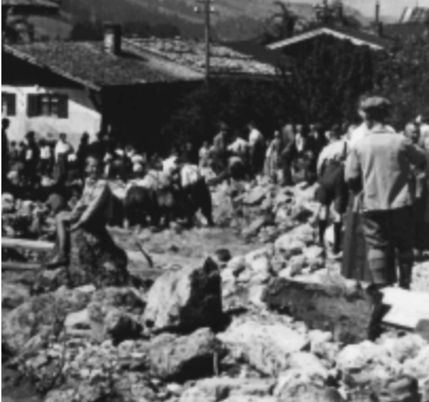
Fig. 3. Photograph of flood damage in Bad Oberdorf from 1924 (M. of Hindelang).
