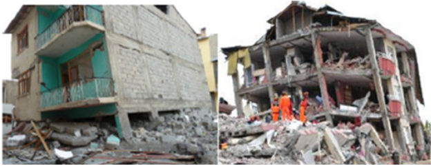
Figure 21. Damage observed in buildings with insufficient lateral rigidity.
