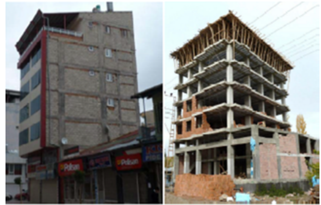
Figure 20. Buildings that do not have adequate shear walls.
