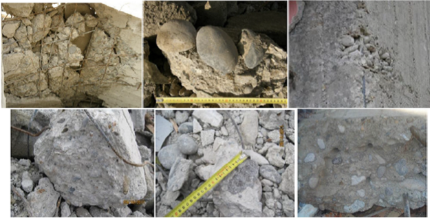
Figure 27. Concrete and aggregate samples in a single-story reinforced concrete building that collapsed in the Van organized industrial site (20) and a concrete cross section displayed in the wreckage (Kizilkanat et al., 2011).
