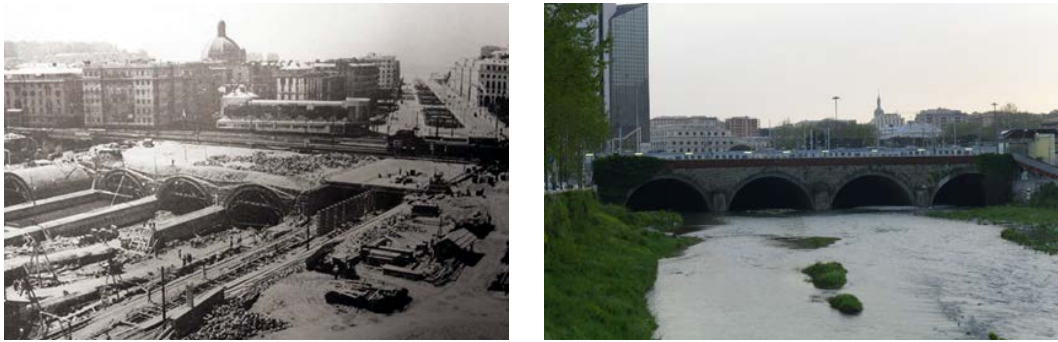
Figure 10. The Bisagno stream culvert during its construction (1930) and in the present day.
