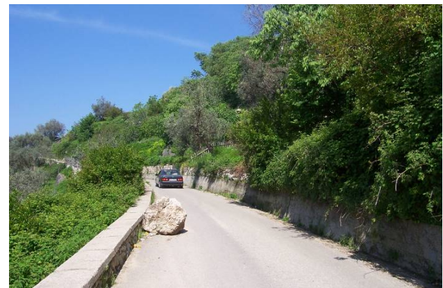
Fig. 20. A limestone block fell on the Kruja urban area during heavy rain in 2010.
