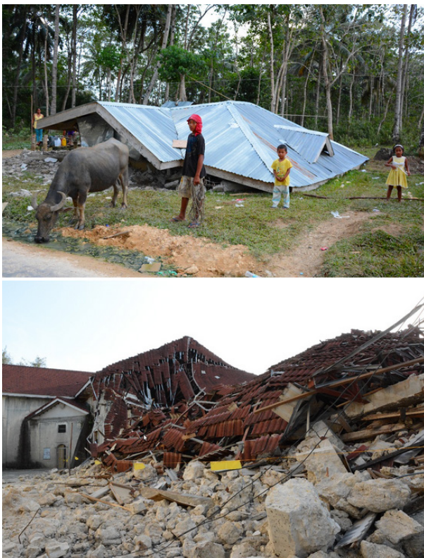
Figure 2. Images of the disaster: top – collapsed house in Sagbayan municipality, Bohol. Bottom – Inabanga church in Bohol. Photo credit: A. M. F. Lagmay (photo taken on 23 October 2013).
