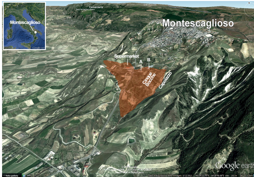
Figure 1. Montescaglioso, southern Italy. The red area shows the area affected by the 3 December 2013 Montescaglioso landslide. Locations of a supermarket (A) and of most damaged buildings (B and C) are shown. (D) and (E) show locations of the Cinque Bocche and Capoiazzo channels. Source of terrain map: Google Earth™.
