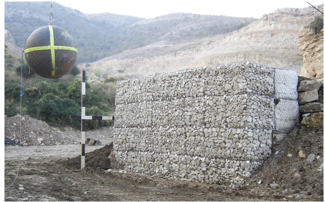
Figure 1. View of the tested embankment, showing the sandwich wall leaned against the levee and the hanging projectile.
