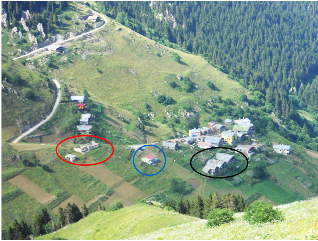
Fig. 5. Damaged school building (red ellipse) and houses (black ellipse) due to the 1981 avalanche; house indicated in blue circle constructed in 2004.
