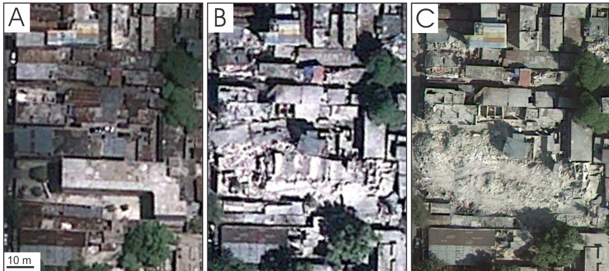
Fig. 2. Neighborhood in Port-au-Prince (Haiti) severely affected by the 12 January 2010 earthquake. Pre-event Geoeye-1 satellite image (26 August 2009; A ), first post-event satellite scene (Geoeye-1, 13 January 2010; B ), and airborne image acquired on 25 January 2010 ( C ). ©Google Earth.
