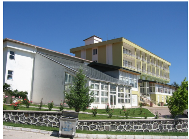
Fig. 8. Building facade and lateral facade (case study 1).
