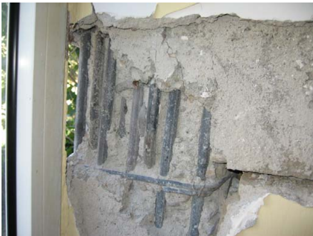
Fig. 12. Utilized rebar (beam-column node of ground story).
