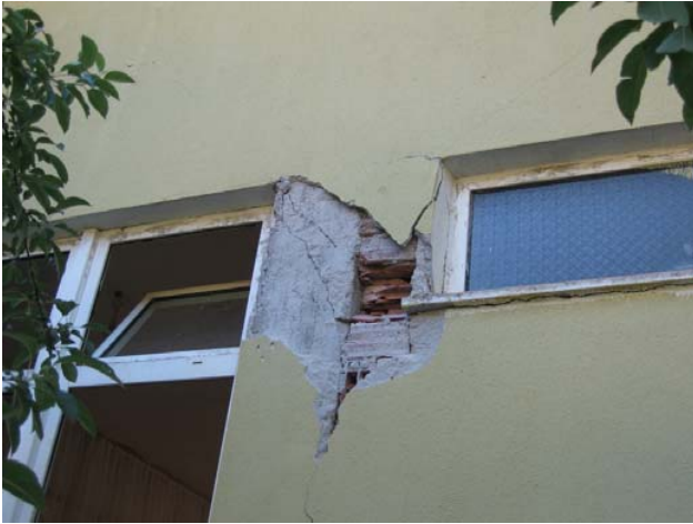
Fig. 11. Shear-column damage.
