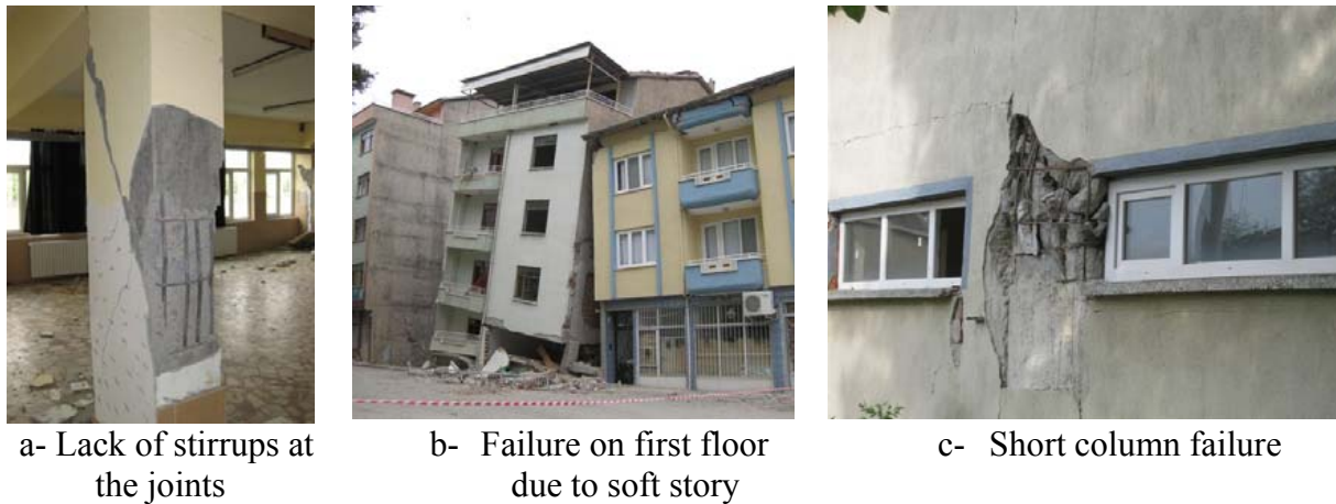
Fig. 6. Three damage types from epicenter region.
