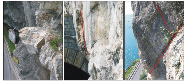
Fig. 3. Examples of unstable blocks impending over the studied road stretch.
