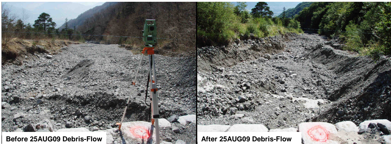
Fig. 7. Photo sequence displaying channel scouring of the August 2009 debris-flow in the main channel of the Manival; views looking downstream.
