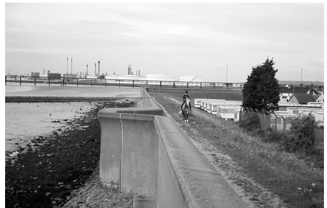
Fig. 10. Improved flood defences built to protect Canvey Island following the 1953 flood. (Source: Baxter, 2005).
