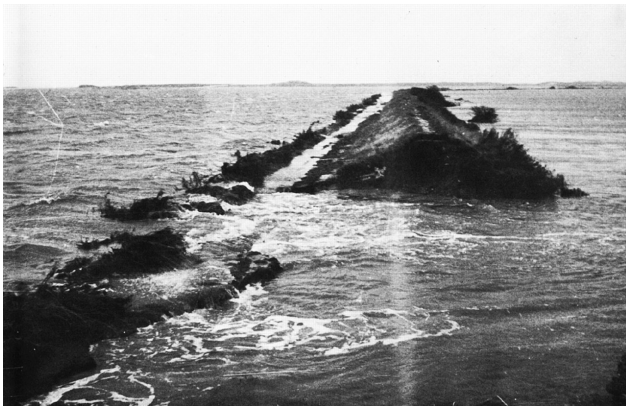
Fig. 2. Typical breach in the flood defences during the 1953 floods. (Sources: Pollard, 1978, and Baxter, 2005).
