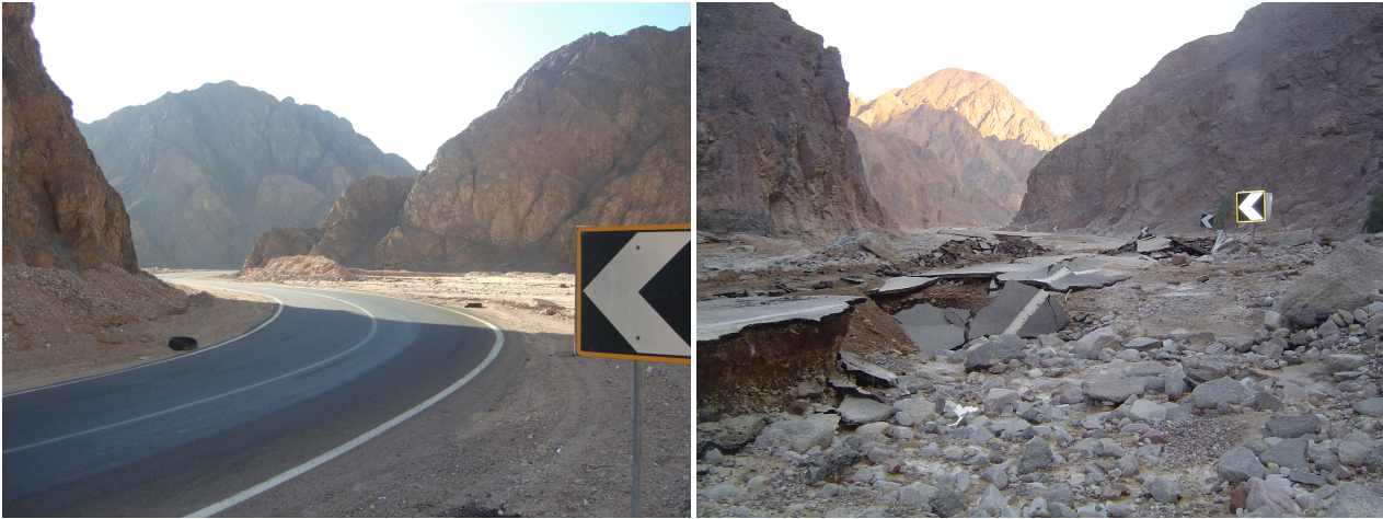
Fig. 4. International road running through the canyon, close to the outlet Wadi Watir. Left: normal state in dry conditions; Right: damage resulting from the flash flood of 24 October 2008.
