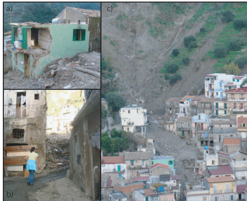
Fig. 4. Examples of the damages caused by one of the seven debris flows that occurred in Giampilieri. In (a) and (b) details of picture (c) are shown.
