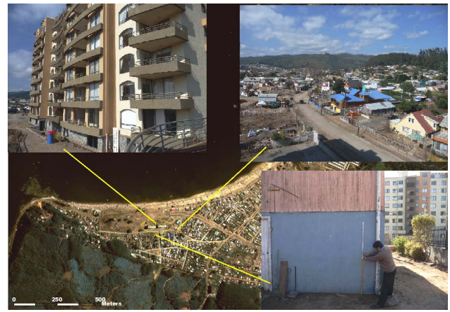
Fig. 2. Location of the ten-story apartment buildings and surrounding houses.
