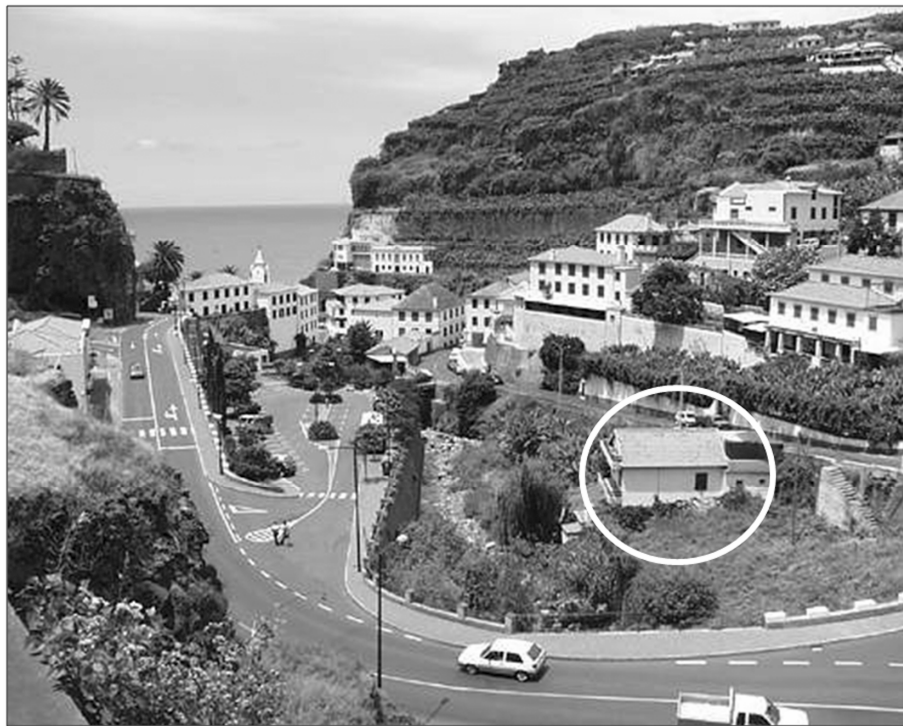
Fig. 9. City of Ponta do Sol: artificial elbow of the course of the “Ribeira do Ponta do Sol” built in the upper part of the city; inside the artificial riverbed a house is located (white circle). Image courtesy of Domingos Rodrigues (Madeira University).
