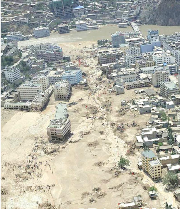
Fig. 12. The devastating amount of sediment and debris transported onto the existing alluvial fan as a result of the major debris flow of Zhouqu, China, 2010.
