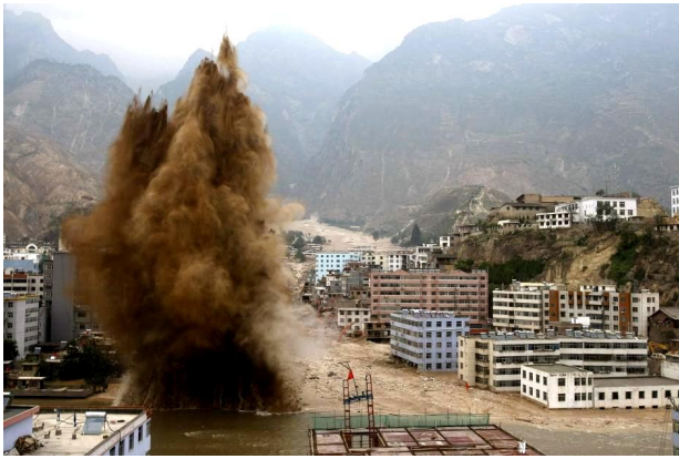
Fig. 15. Breaching of the debris-dams that partially blocked the river, raising the riverbed. After five days, an artificial spillway was completed to successfully release the impounded water.
