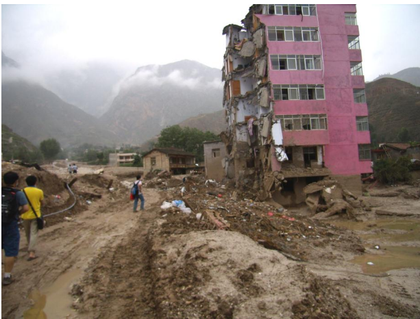
Fig. 13. Apartment buildings in Zhouqu city extensively damaged by the passage of the debris flow front of at least 4 m in height.
