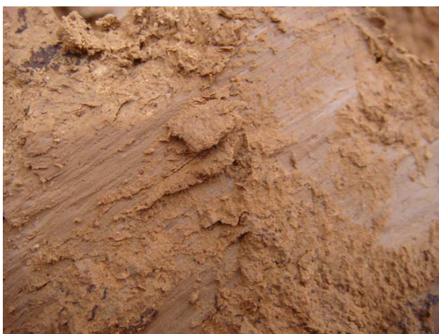
Plate 1. Linear striations of soils along the main sliding surface of the Liujiaquan landslide.
