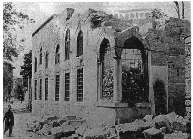
Fig. 5. Another example of damage caused by the 1894 earthquake in Istanbul ( http://www.tarihimiz.net/v3/haberler/genel/tarihte-istanbul-depremleri.html ).
