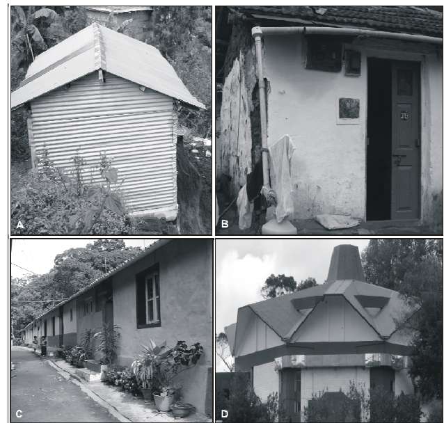
Fig. 6. Building types in the study area. (A): tin shed, (B): brick in mud without column structure, (C): brick in cement with column structure, and (D): reinforced concrete.
