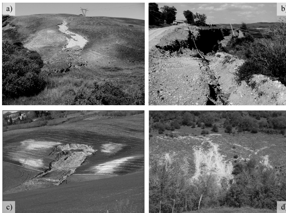
Fig. 5. Examples of the landslide types widespread in the study area: (a) mud flow; (b) earth slump; (c) complex landslide (earth slump evolving into a mud flow); (d) shallow mass movements.
