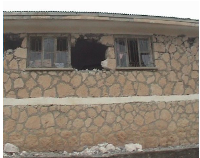
Fig. 8. Short distance between two openings.
