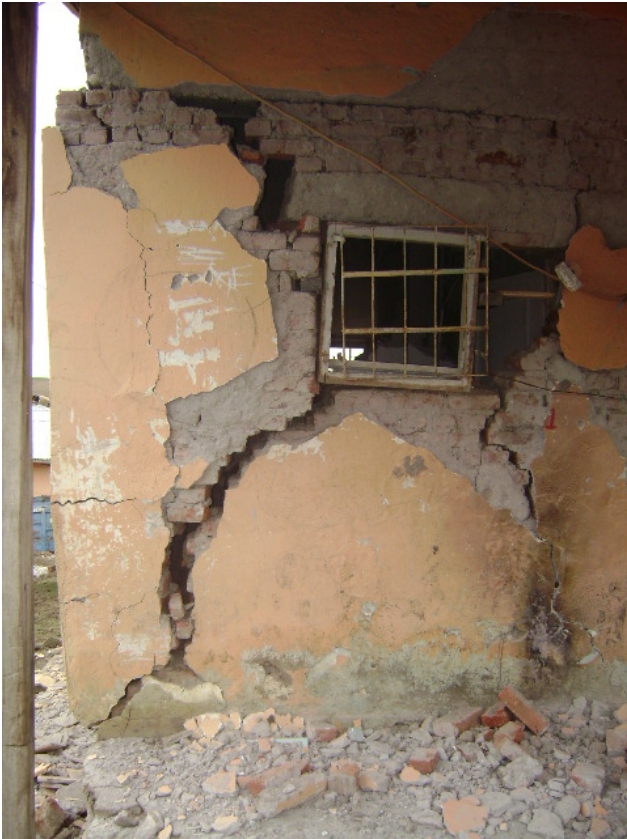
Fig. 9. Wall opening close to the building corner.
