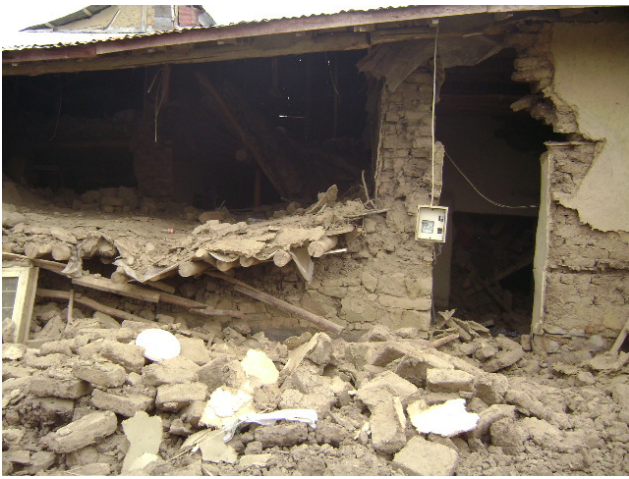
Fig. 5. Heavy roofing with wooden skeleton.
