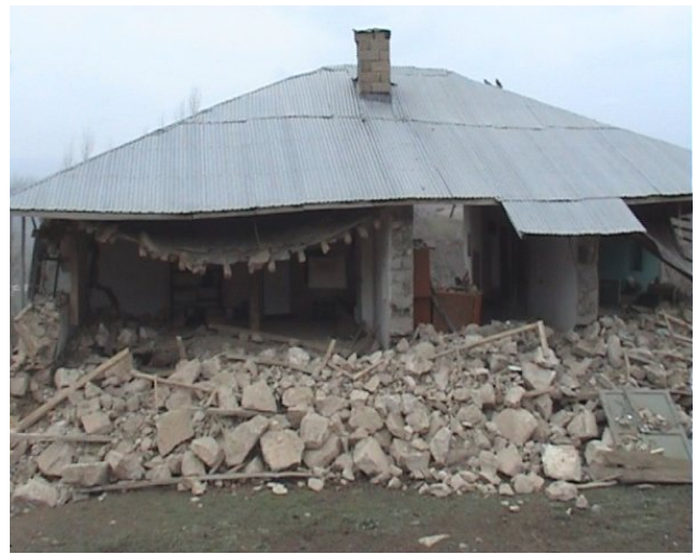
Fig. 7. No connection to partition walls.
