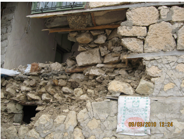
Fig. 6. No interlocking between wall leaves.
