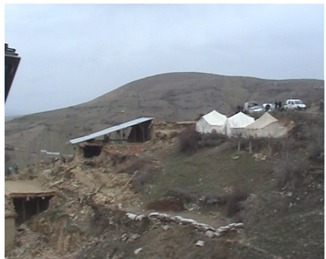
Fig. 11. Damaged buildings on a hill with high slope.
